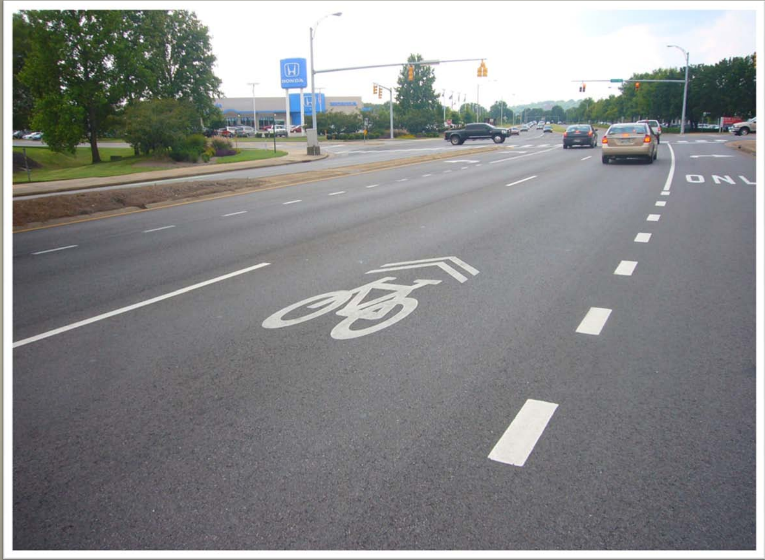
SR-12/ Rosa Parks Blvd. resurfacing project
